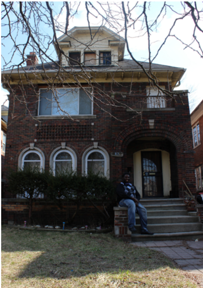
Denzel Donald sits on the steps of his Detroit home. Donald enrolled in WRAP after a broken water pipe in his basement caused escalating water bills.
