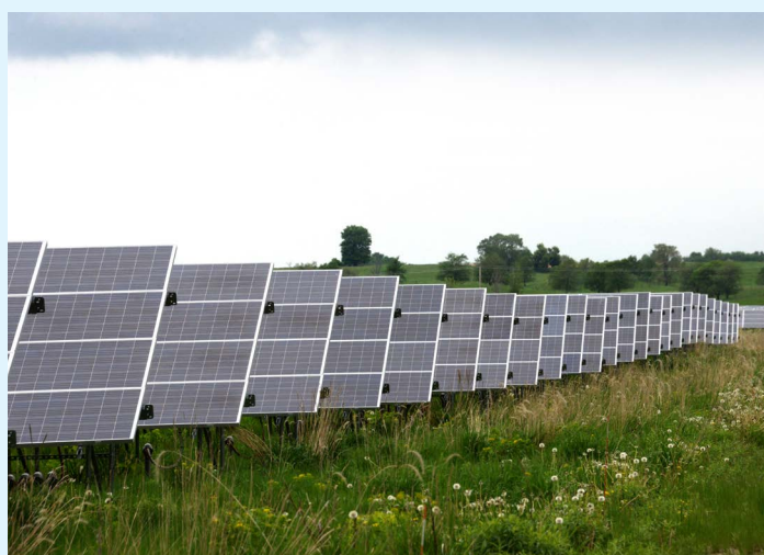
Five-megawatt community solar garden at the Empire Water Resource Recovery Facility. Photo credit: Metropolitan Council
