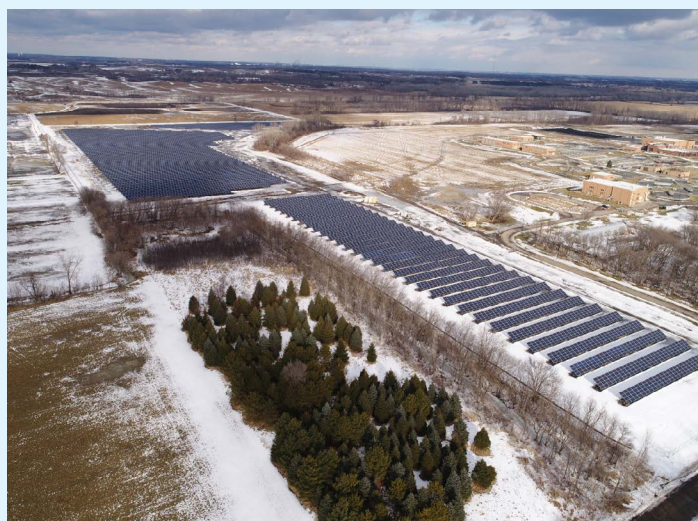
Aerial view of the five-megawatt community solar garden at the Empire Water Resource Recovery Facility. Photo credit: Metropolitan Council
